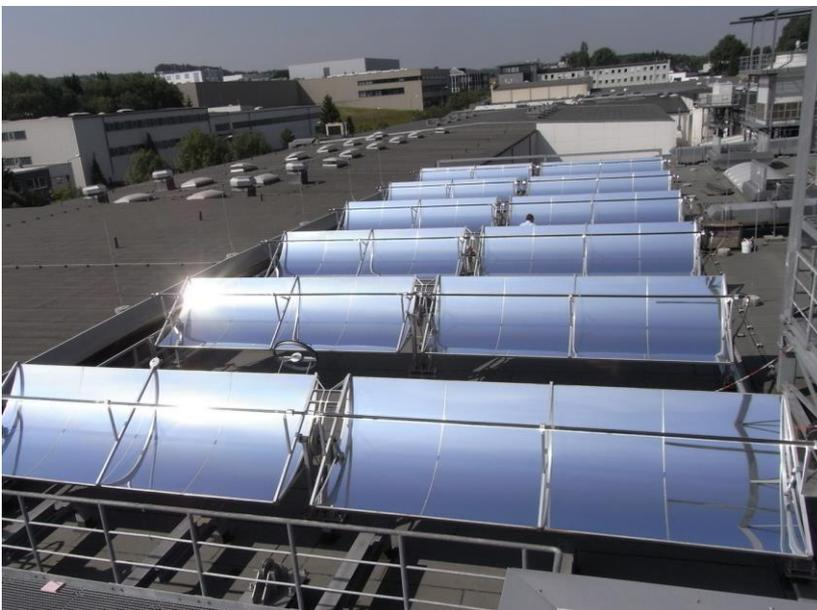
Figure 4: Solitem's 75 kWth Parabolic Trough plant at aluminium surface specialist Alanod in Ennepetal, Germany
