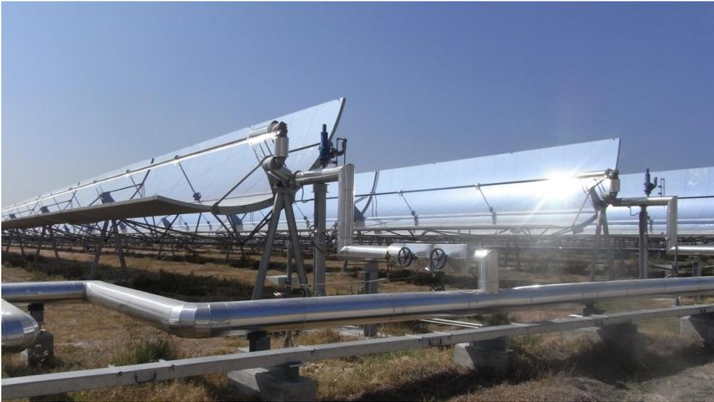
Figure 3: Solarlites Parabolic Trough collectors connected to the hydraulic loop of the 20,8 MWth solar field in Kanchanburi, Thailand [15]
